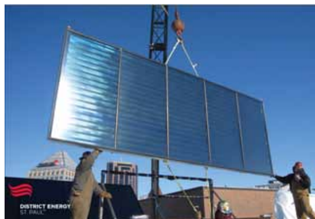
Figure A-94. Sheehy/Amerect installation of Arcon panel (2010).
