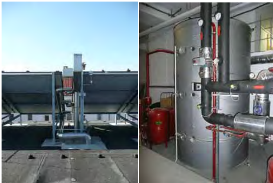
Figure A-48. Collector row piping seen from the backside of first collector row (left side) one of two solar storage tanks (right side).
