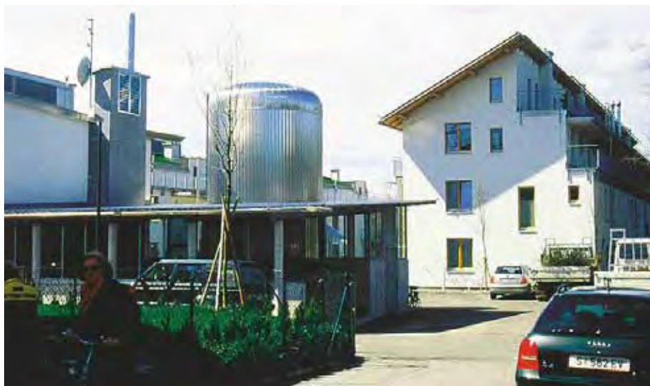
Figure A-7. Part of the 26,420 gal (100 m 3 ) energy storage tank appears from the underground in the middle of the housing estate Gneis-Moos.
