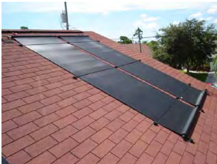
Figure 3.12. An unglazed solar mat-type solar collector made by FAFCO installed on a roof in California.
