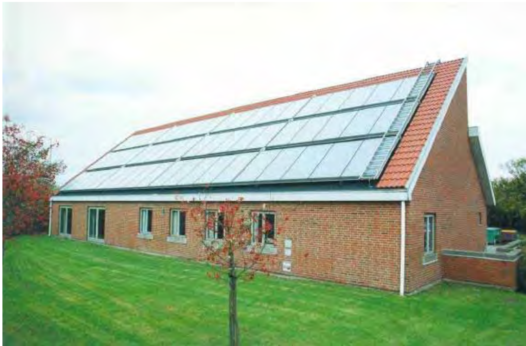
Figure A-26. Service building with collectors.
