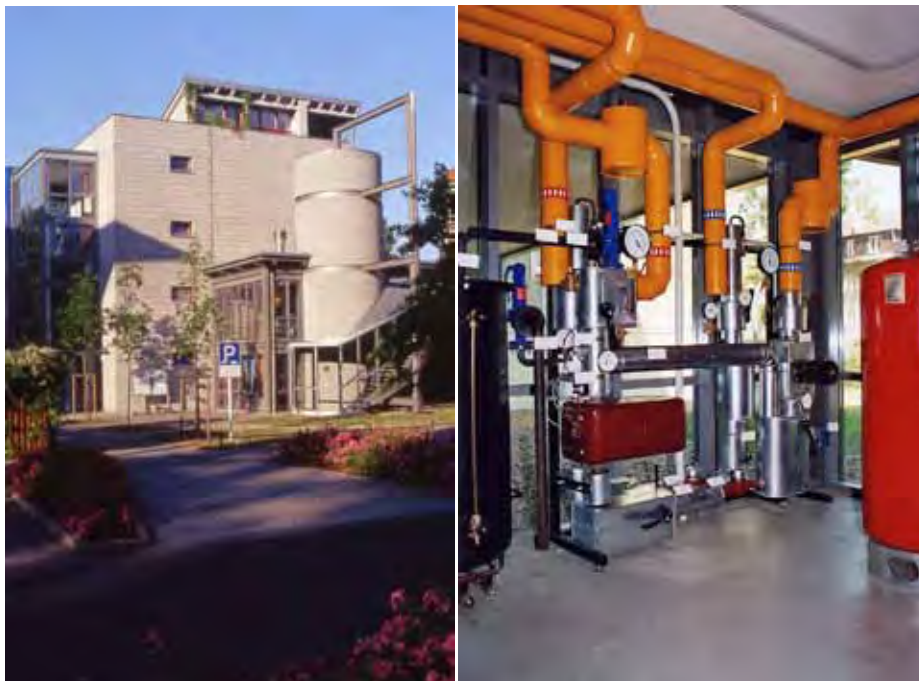
Figure A-55. Heating central with in-housed solar storage tank (left), collector loop flat plate heat exchanger (red box) with piping (right).
