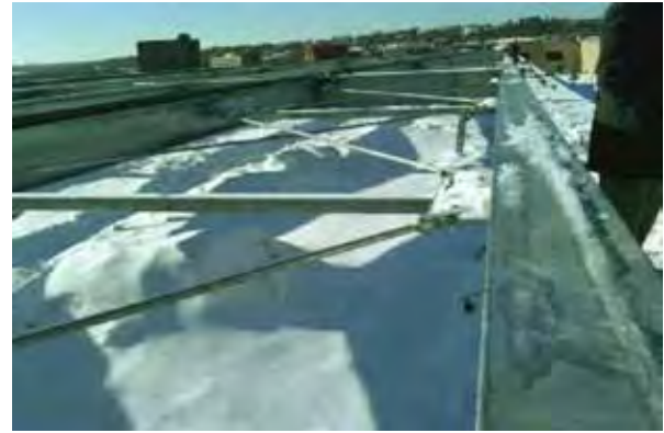
Figure A-96. Steel bracing.
