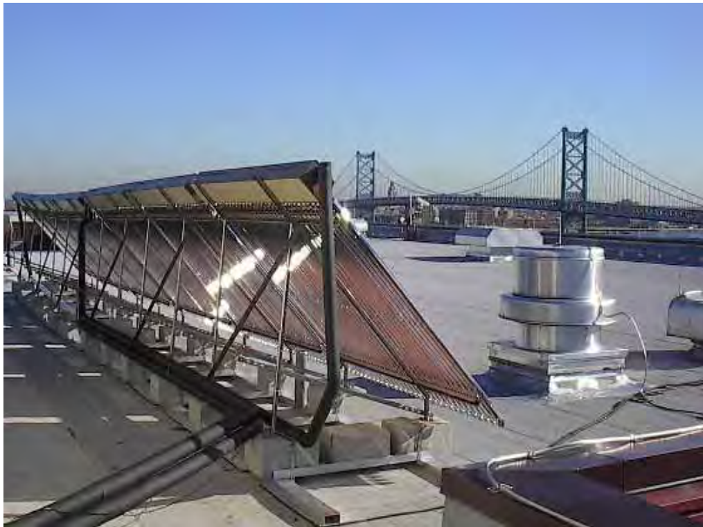
Figure A-106. The solar water heating system installed on the SSA building is a re-circulation loop system using 360 evacuated tube collectors that cover 54 m 2 gross area.
