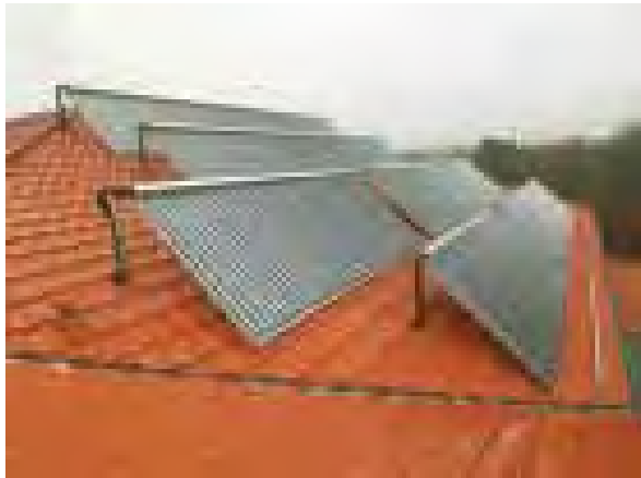
Figure A-121. View of solar panels installed at AWO Rastede, Oldenburg, Germany.
