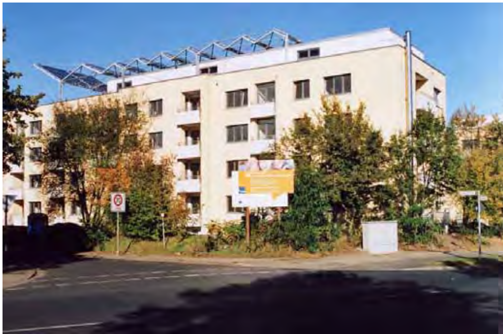
Figure A-73. Front view of the apartment building with nine collector rows on a flat roof.
