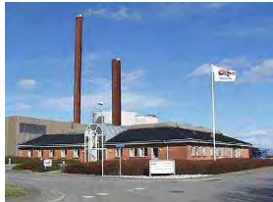
Figure A-33. The district heating plant at Brædstrup, Denmark.
