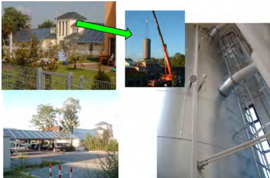
Figure A-41. District heating Speyer “Old slaughterhouse” 5866 sq ft/26,400 gal (545 m 2 / 100 m 3 ).
