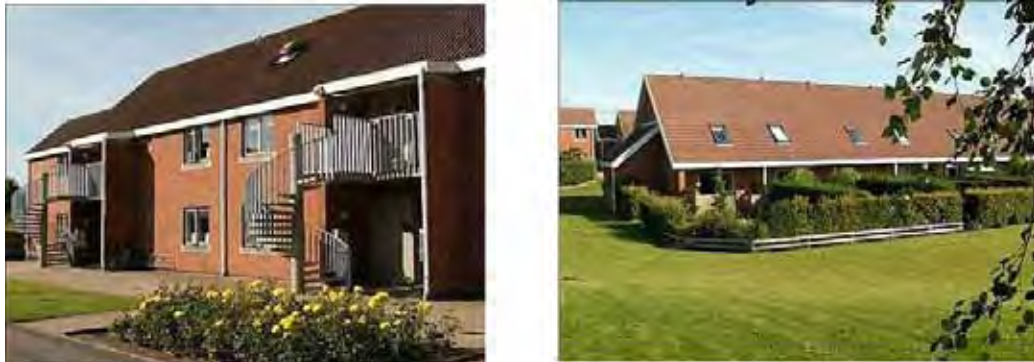
Figure A-25. Different types of buildings in the complex.
