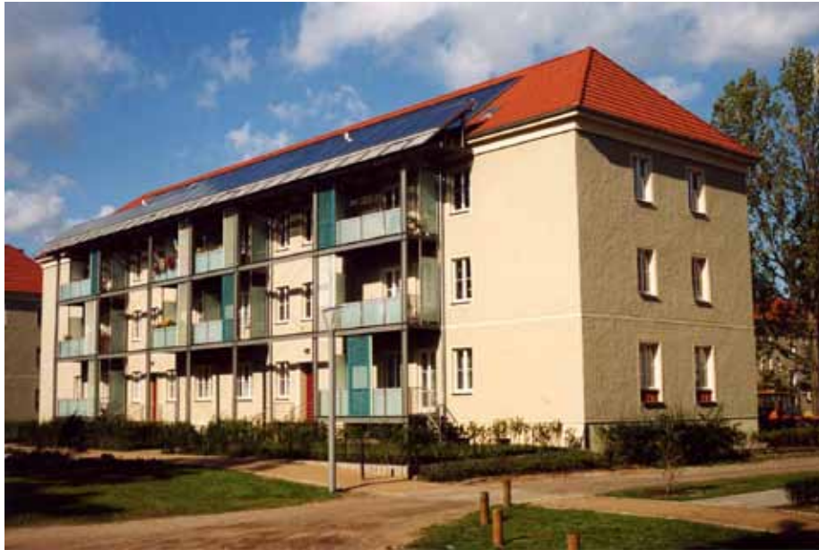
Figure A-54. One of five collector areas partly roof-integrated.
