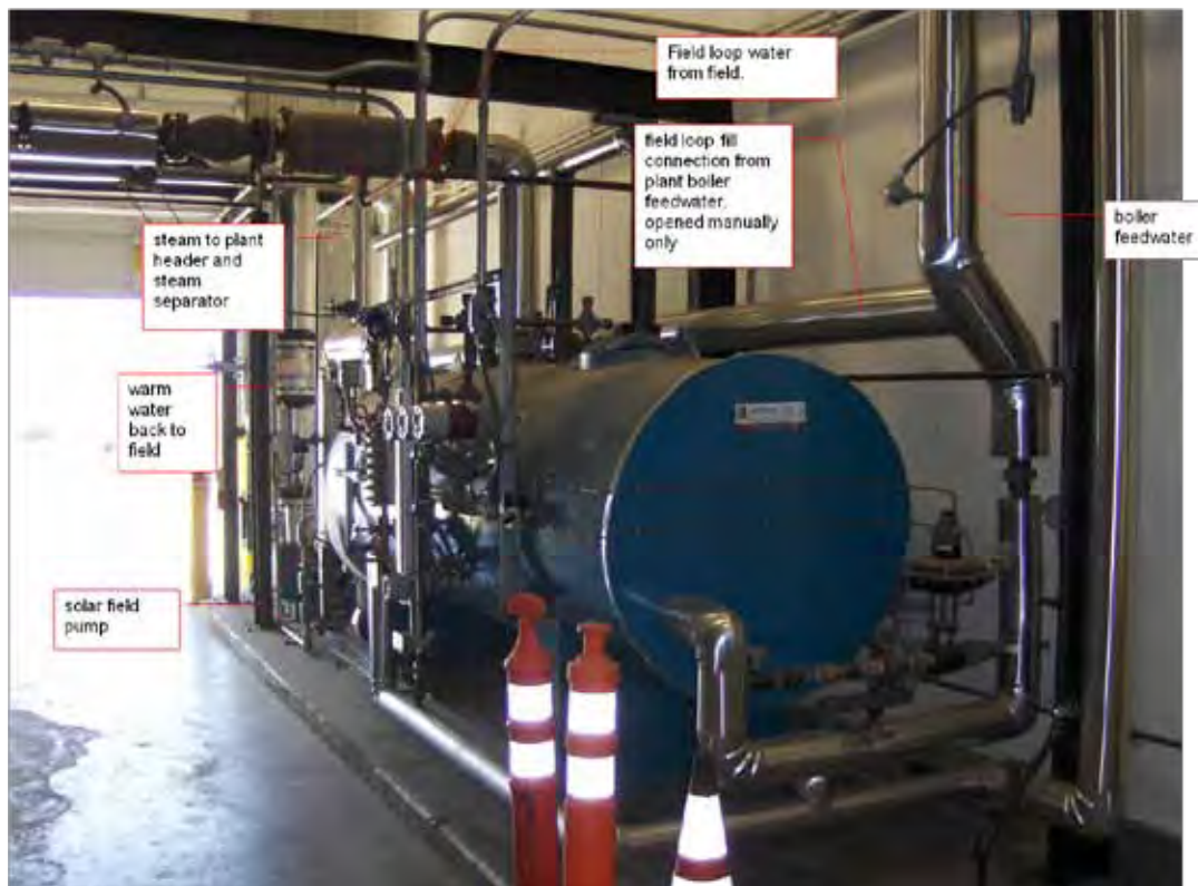
Figure A-128. Components of a 54,000 sq ft (5022 m 2 ) solar industrial process heat plant at Frito Lay Modesto CA, including an unfired steam generator, pump, and controls.
