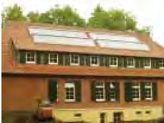
Figure A-116. Solar panel installation at Wohnheim Langendamm, Nienburg, Germany.
