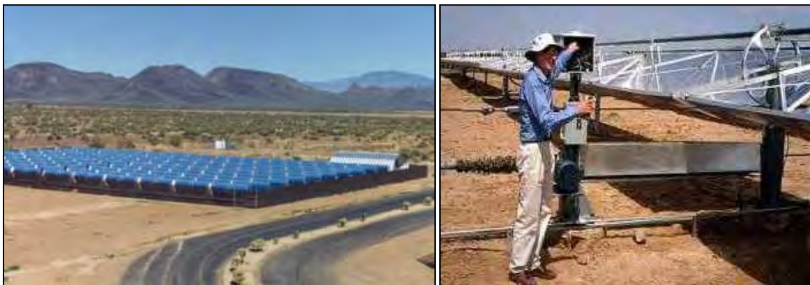
Figure A-125. Solar field of collectors at the Phoenix correctional facility (left); close-up of a row of parabolic collectors at the prison (right).
