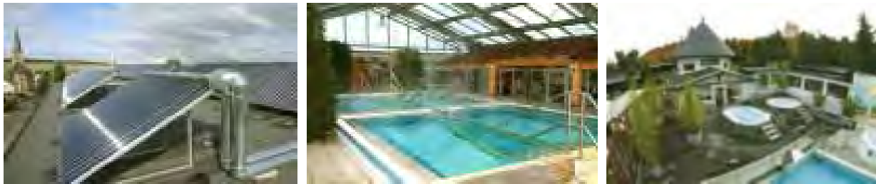
Figure A-114. Solar system at Panoramasauna, Holzweiler, Germany.
