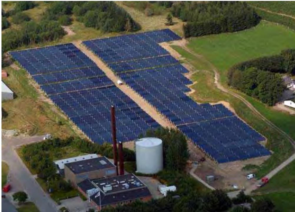
Figure A-32. Aerial image of the district heating plant of Brødstrup and the solar collector field.
