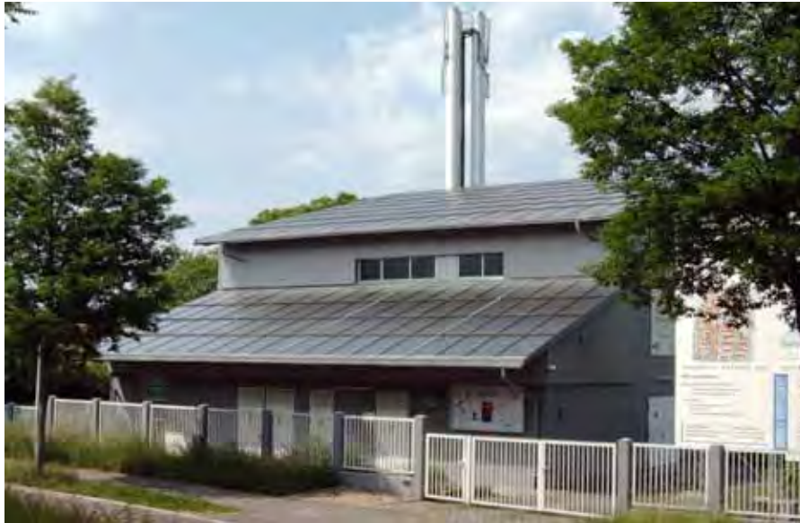
Figure A-63. Front view of the heating central with two roof-integrated collector areas.
