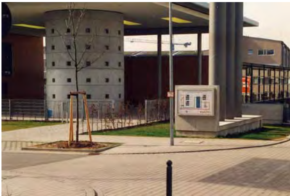
Figure A-81. Solar storage tank encased in a concrete structure and the stacks from the heating central.
