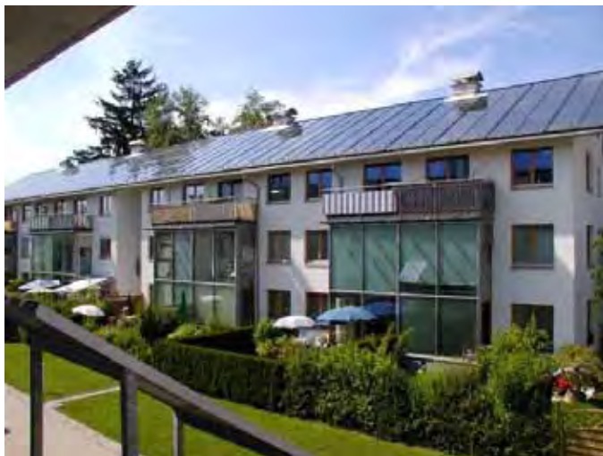
Figure A-2. South oriented glazed façade with greenhouse for passive solar heating.
