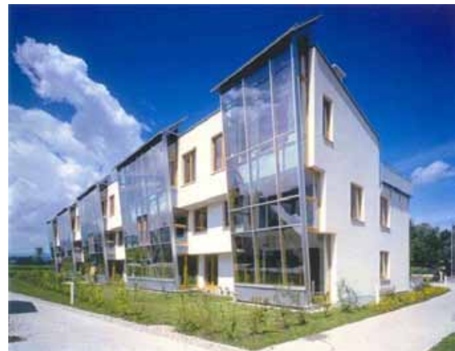
Figure A-2. South oriented glazed façade with greenhouse for passive solar heating.
