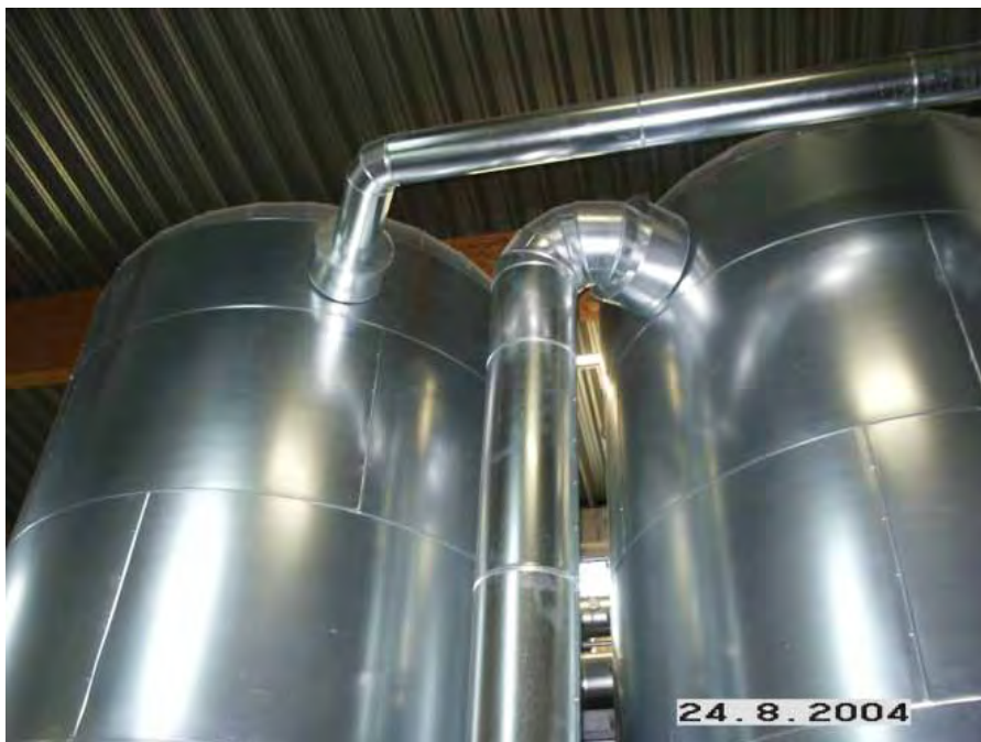
Figure A-64. Solar storage tanks.
