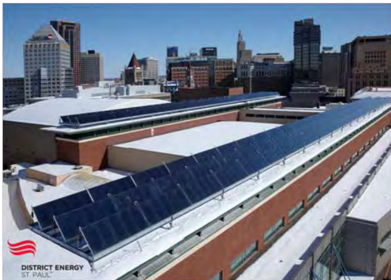
Figure A-86. Aerial view of solar district heating installation at Saint Paul, MN.
