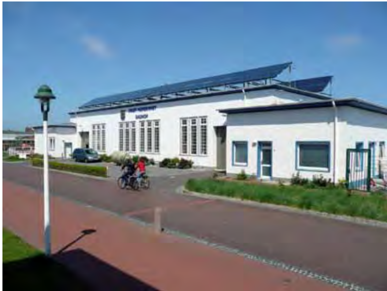
Figure A-47. Front view of the heating central with two collector rows on a flat roof.
