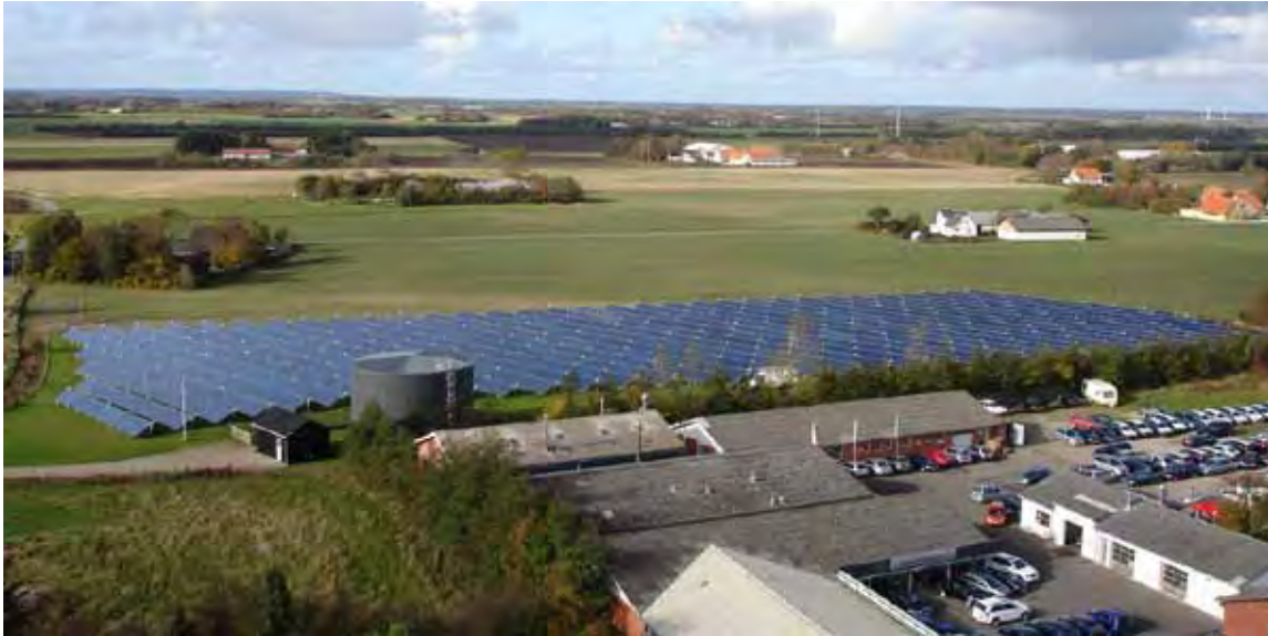
Figure A-20. Aerial picture of the district heating plant of Ulsted and the solar collector field.
