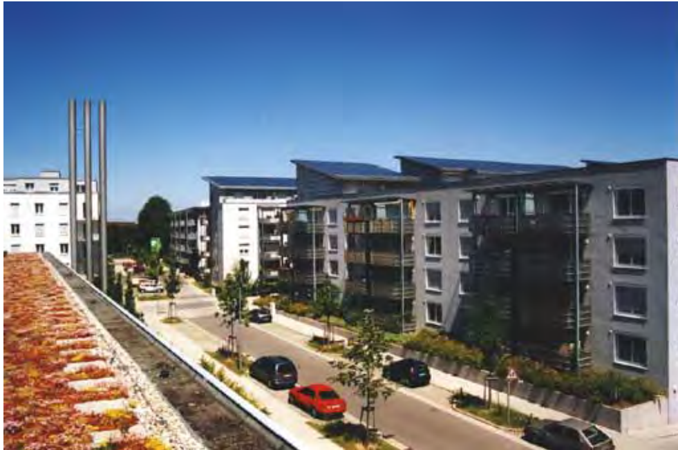
Figure A-80. View from the heating central to some of the buildings carrying a roof-integrated collector area.
