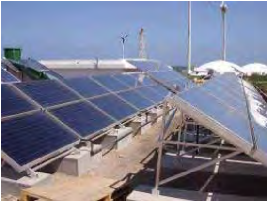
Figure 2.10. Flat plate collectors on mounting construction.
