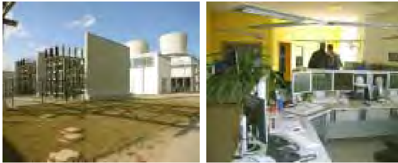
Figure A-119. View of solar system at Kraftwerk, Halle, Germany.
