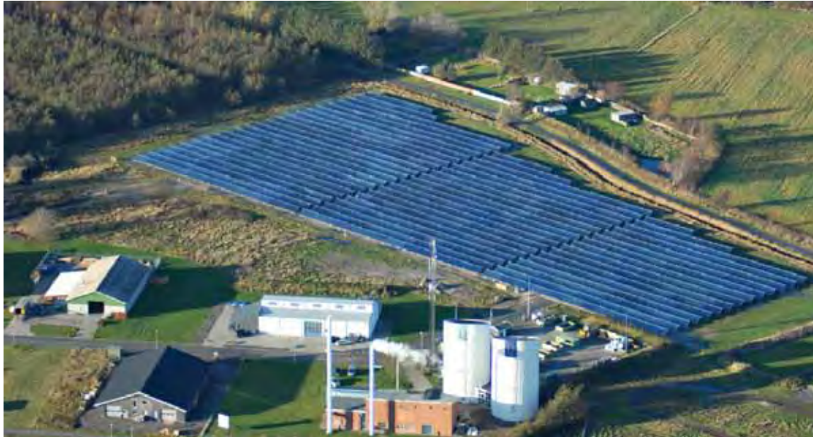
Figure A-22. Aerial image of the district heating plant of Strandby and the solar collector field.
