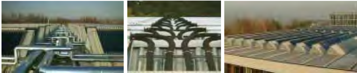
Figure A-110. Solar cooling plant at Festo, Esslingen, Germany.
