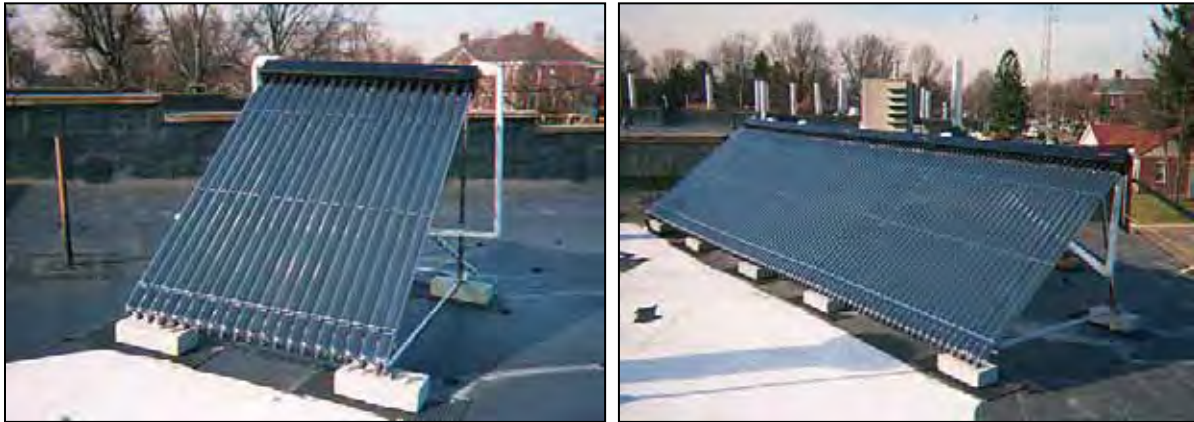
Figure A-105. Evacuated tube collectors installed on the EPA lab in New Jersey.
